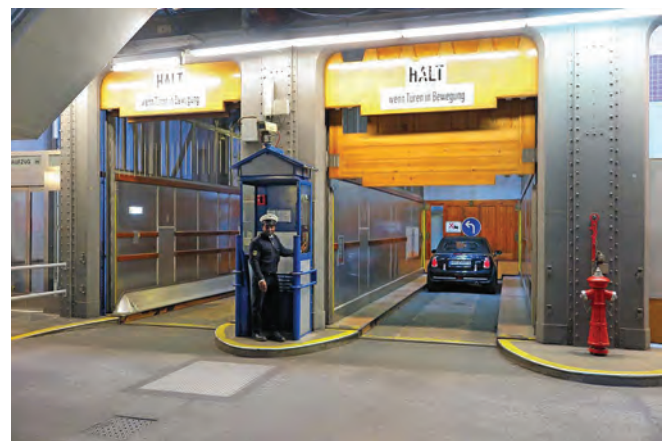
Our guide Mr Salam operating one of the four Old Elbe Tunnel vehicle lifts
